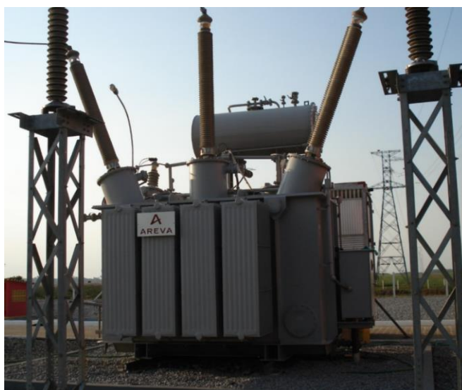
Figure 128: Example of three phase iron core shunt reactor
